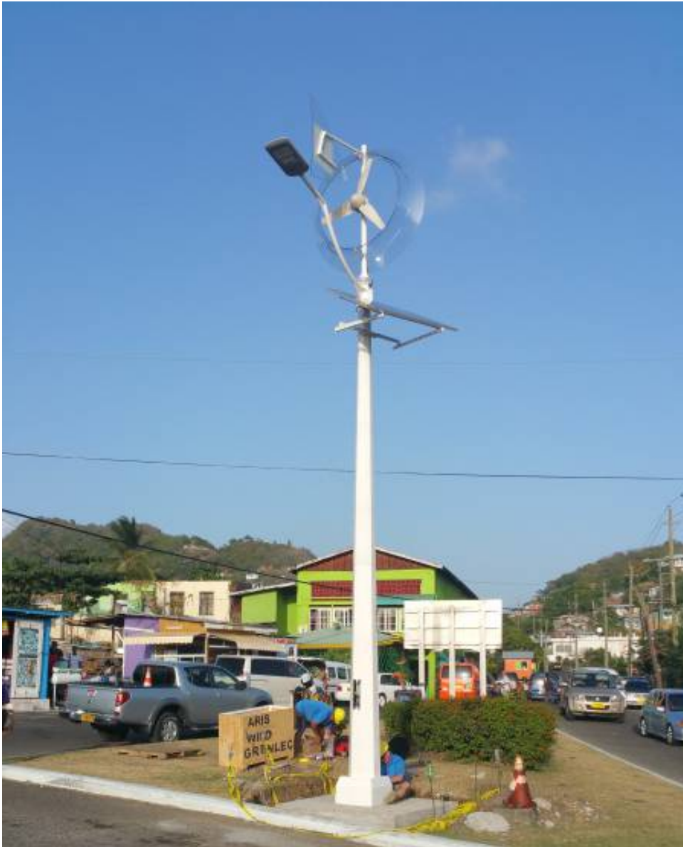
Team Installing Street Light Powered by Wind and Solar Technology
