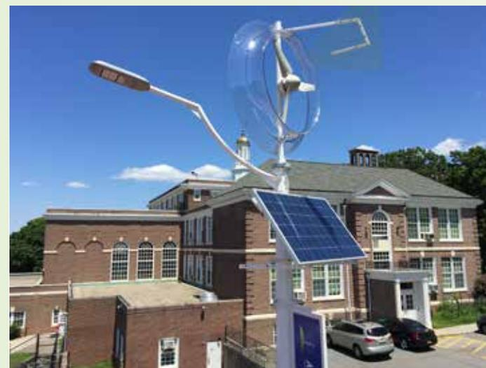
Solar power generation coupled with an advanced wind turbine trickle charge batteries day and night to reliably power lighting and auxiliary power loads.
