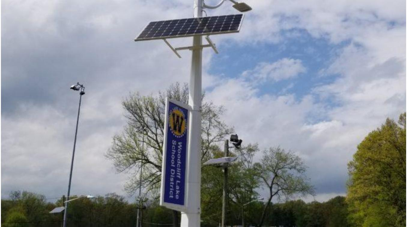
A BRIGHT IDEA! Woodcliff Middle School's new renewable-energy remote power unit, installed on Earth Day, has a wind turbine, a solar panel, and an LED lamp. And it'll charge your phone.
